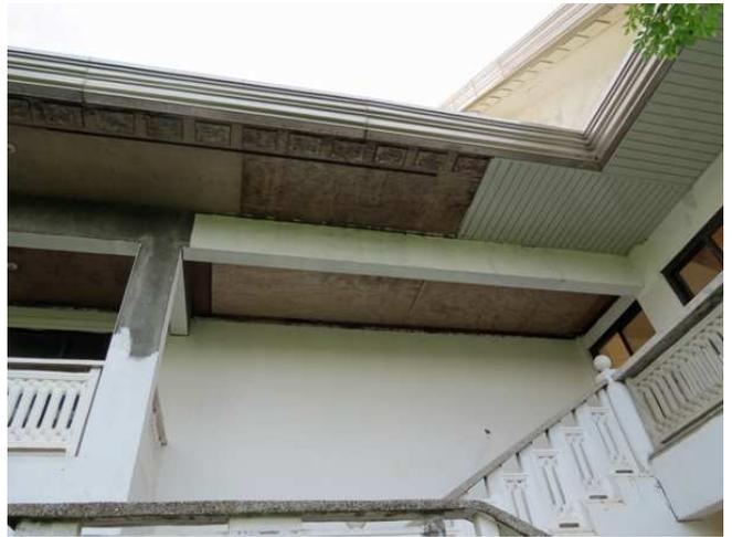
This shows the eaves where we have replaced some rotting wood with steel. This needs to be done all the way around the other 90% of the house.
